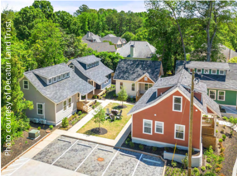
Decatur, GA Cottage Court
